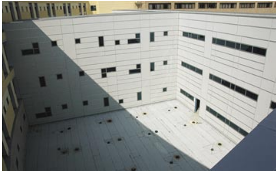
An open courtyard on the building's fourth floor. The courtyard will eventually be a serene place for visitors to sit, with landscaping and comfortable benches.
